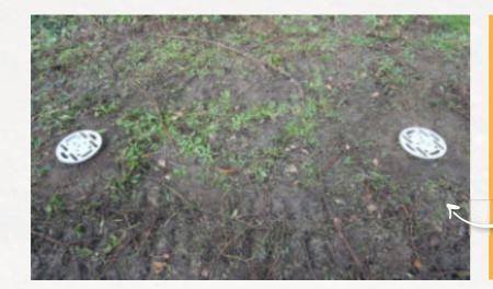
Install 2 ground screw foundations with a centre-to-centre distance of 1300mm. Make sure the flange plate protrudes about 2cm above ground level.
